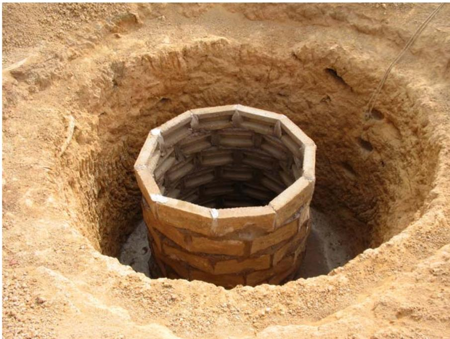
Figure 5: Dutch bricks casing on the Kodougouni well
